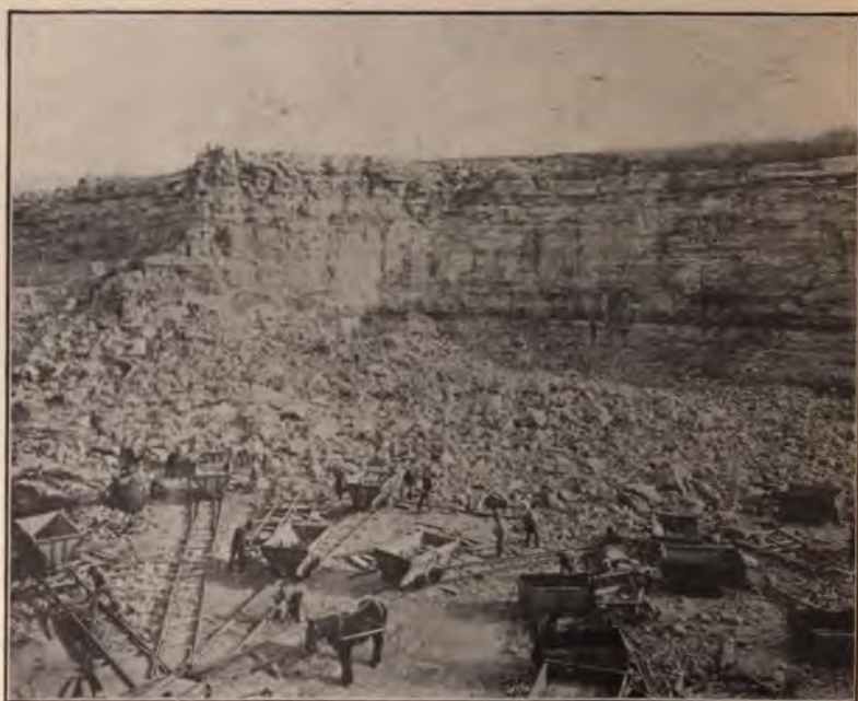
Fig. 55.—Quarry showing Result of Blast.
